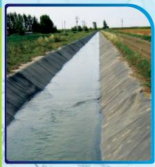
Water is in high demand for irrigation in most of the agricultural areas as the required amount of water is not available naturally. To reduce these problems, canals have been constructed so far to carry water where it is needed. HDPE Geomembrane has been used as a water canal liner to control leakage and is an effective alternative to more traditional lining methods such as concrete and compacted soil.
