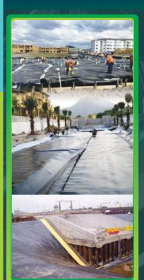
Macro HDPE Geomembrane can be used as a water proofing membrane which can be laid on a surface. Doesn't let water out of it. It can be laid under structural slabs, foundations, flat roofs and finishing tiles. Ensures that water does not seep into the structural slab.
