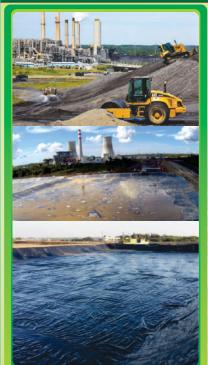
The Boiler Ash is collected from the boiler's hopper precipitator fly ash from the electrostatic precipitator hoppers. This is mixed with water to make a suspension, which is pumped to the ash pond. Macro HDPE Geomembrane provide perfect lining for the ash ponds.
