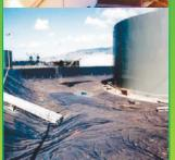
In case of leakage, the secondary anti-seepage layer can play a temporary anti-seepage role. For the period before the leachate is discharged, a second anti-seepage layer can prevent leachate from penetrating the ground. In addition to anti-seepage, this guide also gives ample time for the drainage system to play a role.
