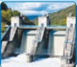
HYDRO ELECTRIC POWER
